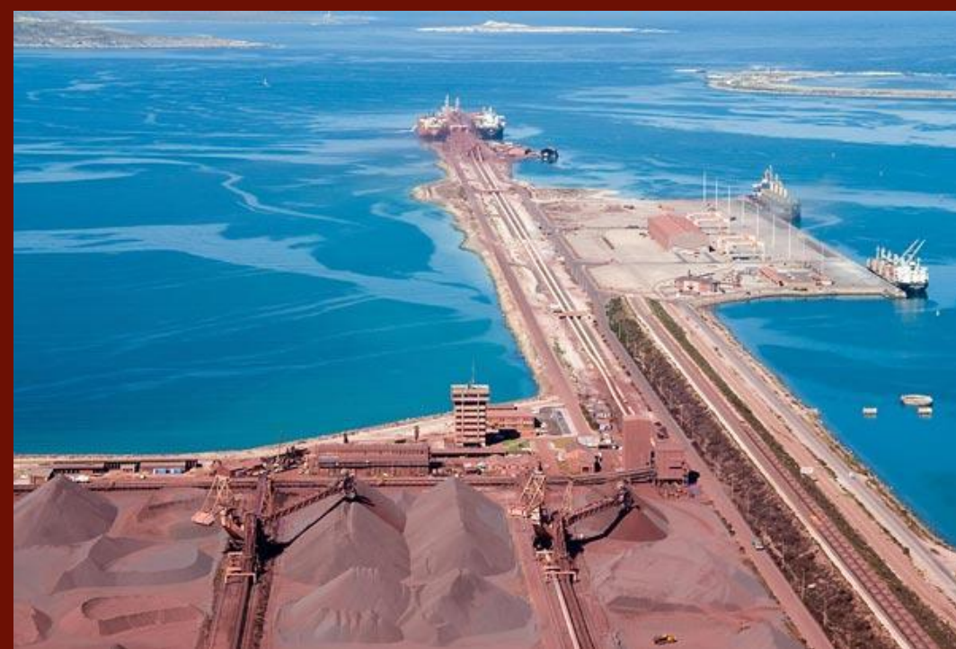
Fig 1: Saldanha Bay Port Terminal
