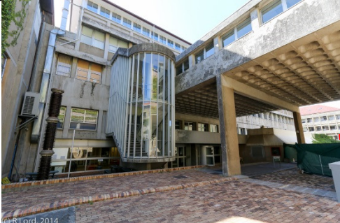
Level 3 (glass house) entrance to Menzies
