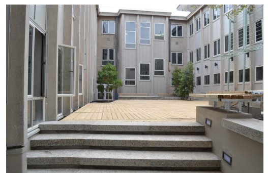
New Courtyard area of Centlivres Building
